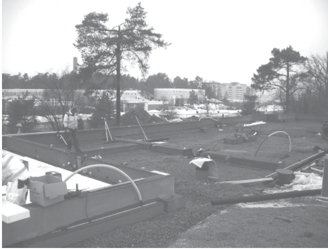
Figure 5.27 The foundation for DLL is built with prefabricated concrete elements.
