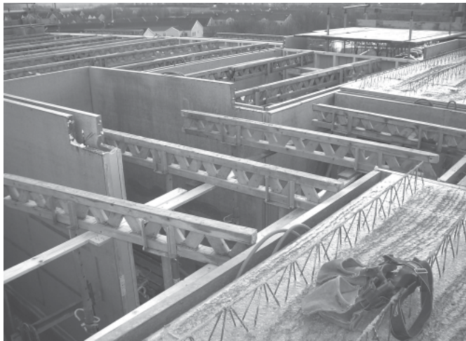
Figure 5.15 The structural frame of concrete elements is assembled at the site.
