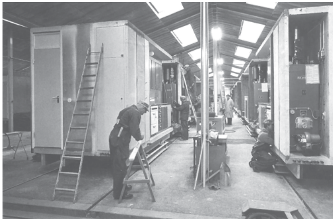
Figure 3.8 A prefabricated kitchen in a volume element during the 1960s 162 .
