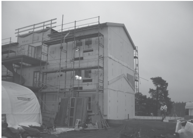
Figure 5.8 The volume elements assembled at the building site.
