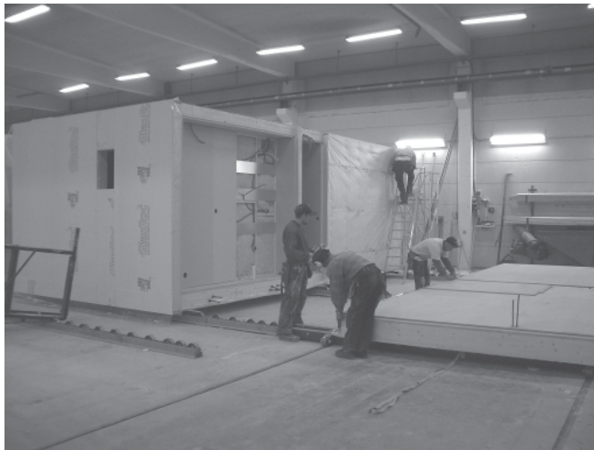
Figure 5.3 Floor and wall elements are pre-assembled to volume elements.
