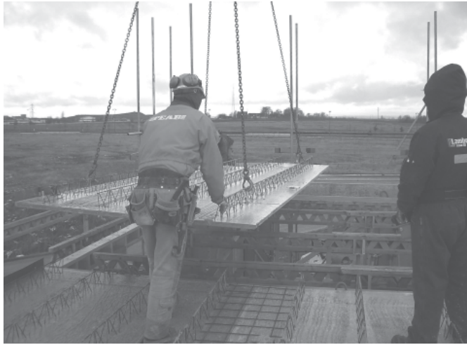
Figure 5.14 Assembly of concrete elements.
