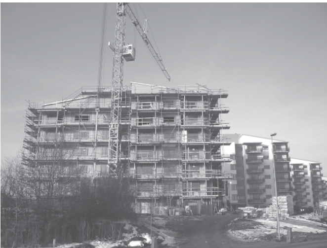
Figure 5.20 Houses of the Solfångaren project.
