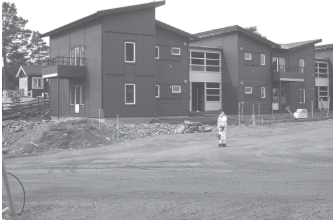
Figure 5.31 One of the DLL houses of the Älta project.
