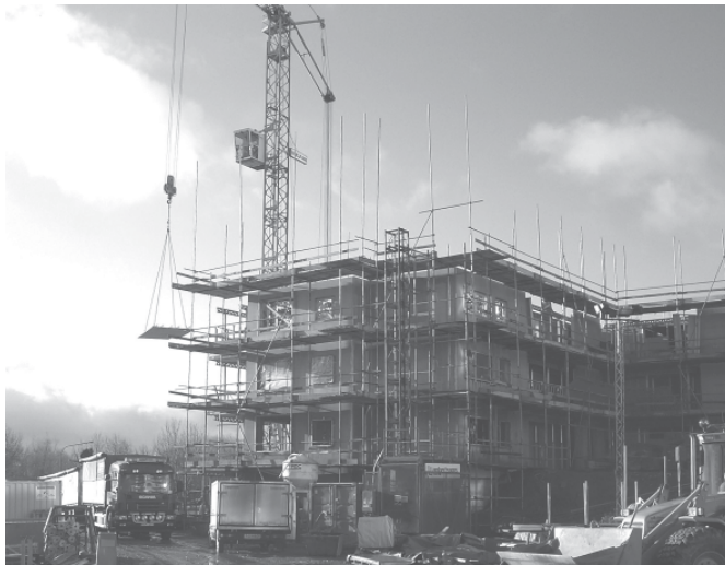
Figure 5.13 One of the apartment houses of the Solfångaren project, based on an open building system.
