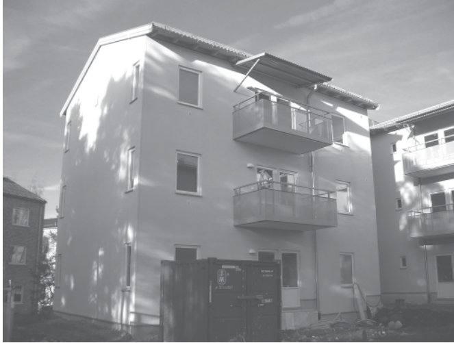
Figure 5.11 One of the finished houses in the Svedmyra project.
