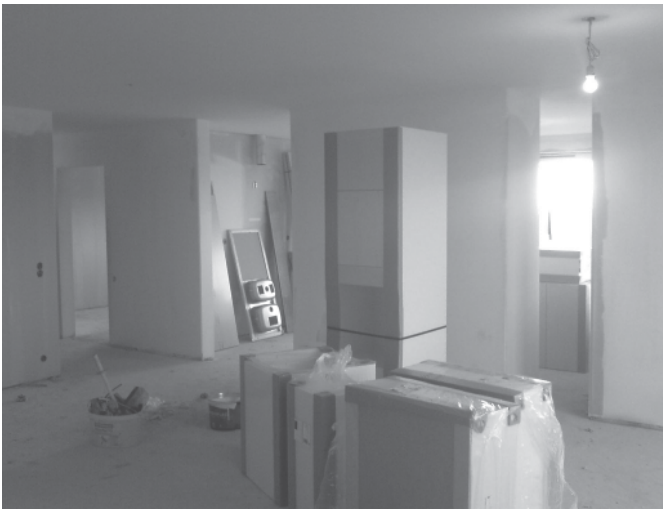
Figure 5.18 Kitchen equipment before assembly in an apartment.
