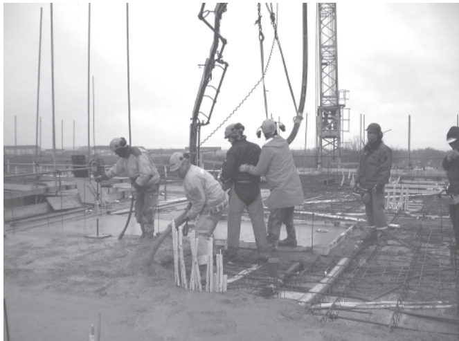
Figure 5.17 The slabs are casted with concrete.
