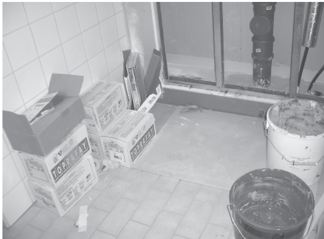
Figure 5.10 Complementing work with a bathroom wall, at the building site.
