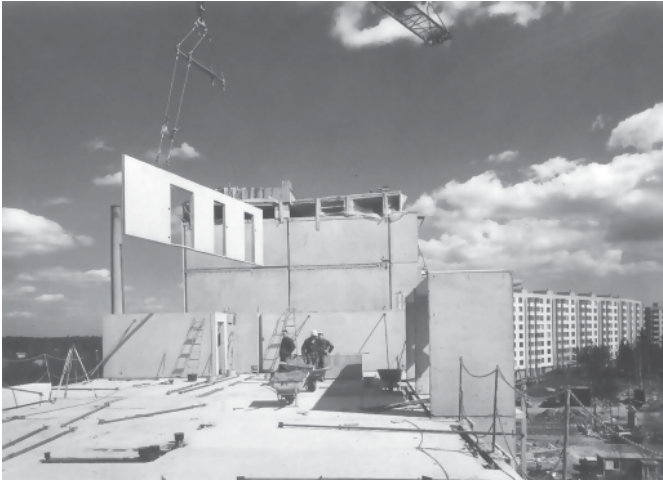
Figure 3.7 Building with concrete elements during the so called Million Programme 144 .
