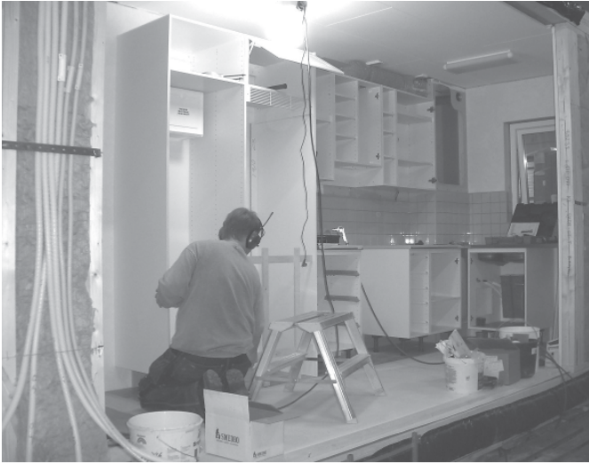
Figure 5.30 All kitchen equipment is pre-assembled in the volume element, at the factory.
