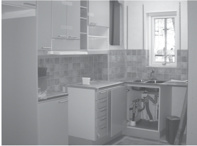
Figure 5.29 A kitchen in a DLL-apartment, ready for installation.
