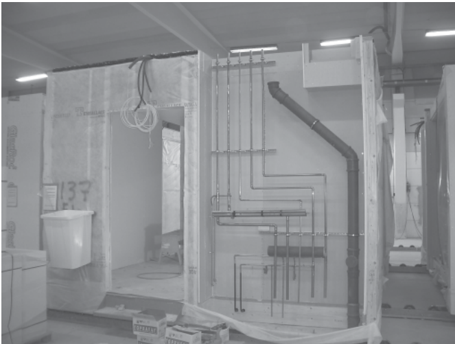
Figure 5.5 Installations in a volume element at the factory.
