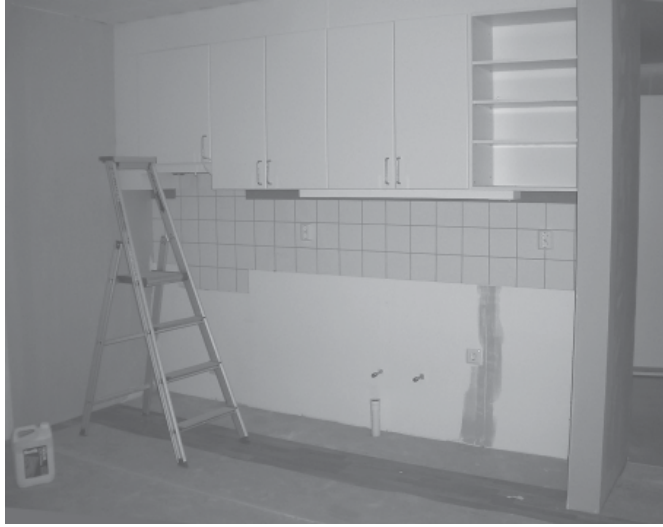
Figure 5.9 Complementing work with the kitchen equipment, at the building site.
