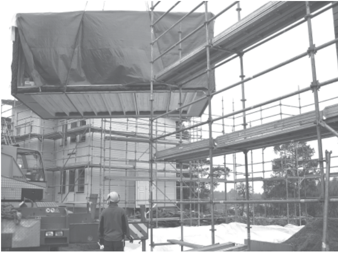
Figure 5.28 A volume element is being assembled at the Älta project.
